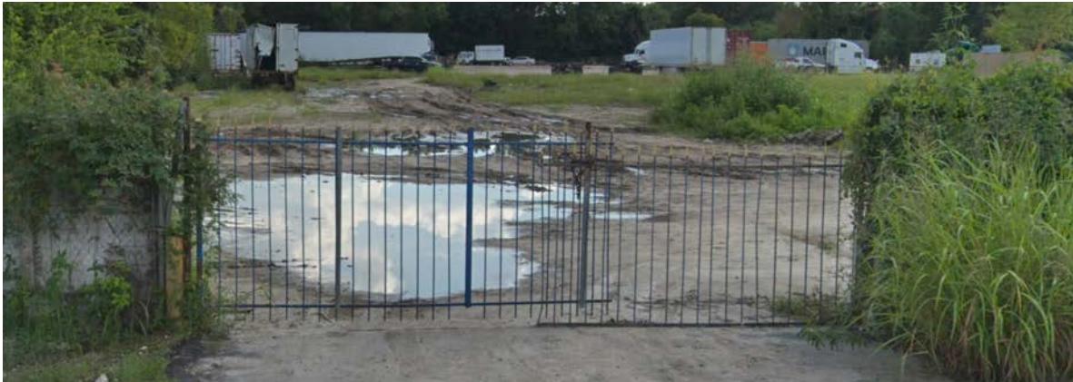
Truck parking on mostly mud and grass surfaces; puddles indicate a lack of grading and draining
