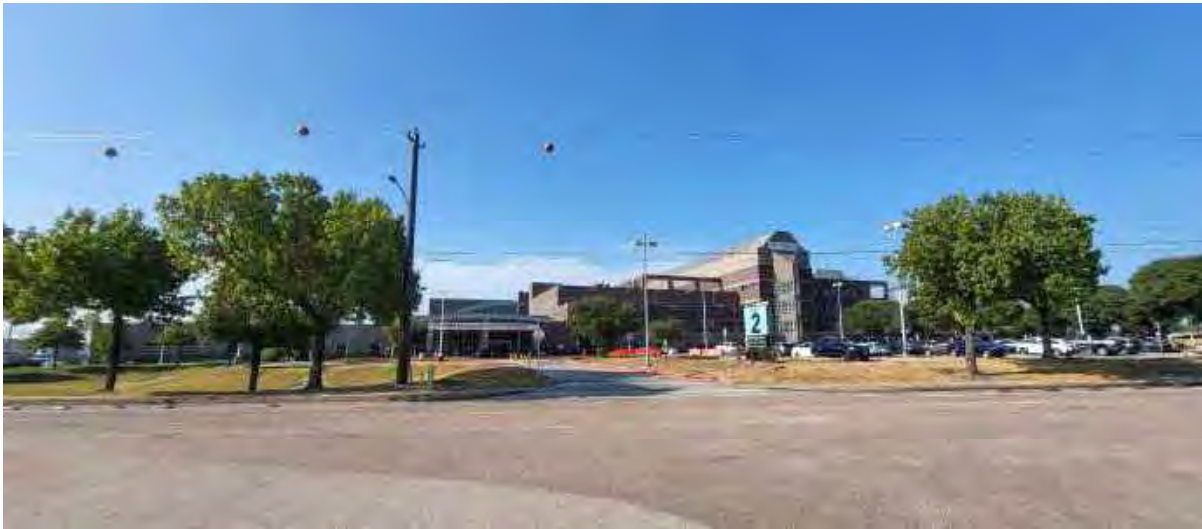
Figure 5 – LBJ Hospital – Facing S from Kelley St.
