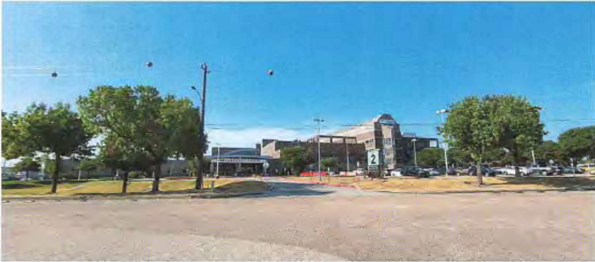
Figure 5 – LBJ Hospital – Facing S from Kelley St.
