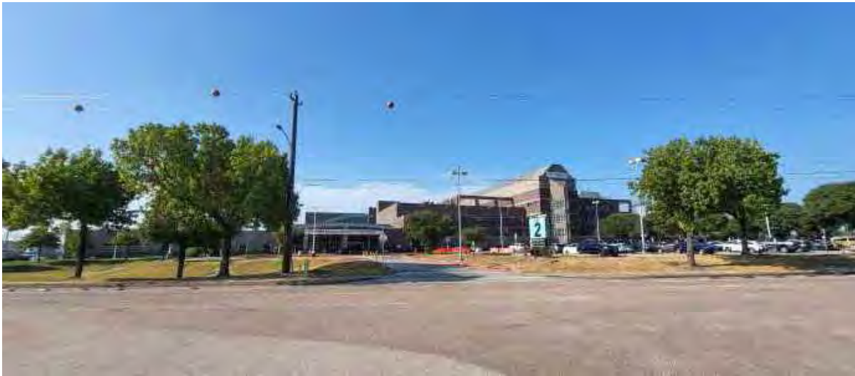
Figure 5 – LBJ Hospital – Facing S from Kelley St.
